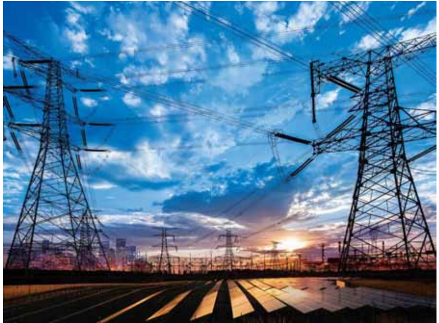
Integration of electricity from renewable energy sources into the grid will be a key challenge for India.
