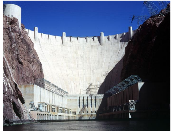
Hoover Dam and Powerplant. (Source: US Bureau of Reclamation, Photo C45-300-021359)
