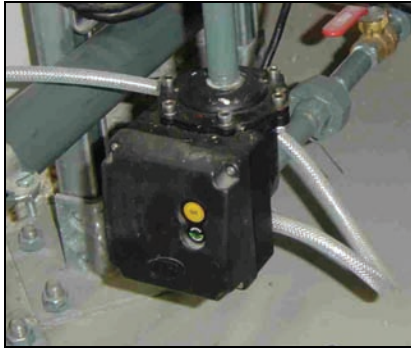
Figure 14 - Example of Zero Air Loss Drain
